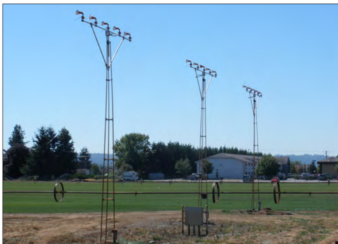
Arlington Municipal Airport leases its RPZ for landscaping business, production of sod.
